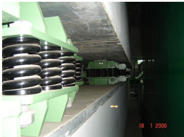
Spring elements between upper and lower decks
