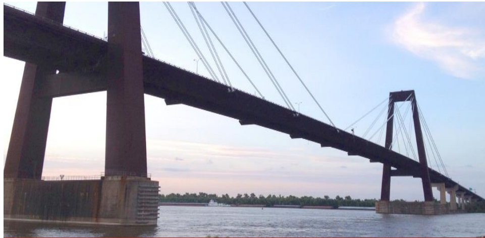
Repair of Hale Boggs Memorial Bridge (Canada)
