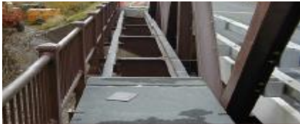
Repair of the Warren Farm Bridge in the village of Wellsburg, Chaemooon county, New York (USA)
