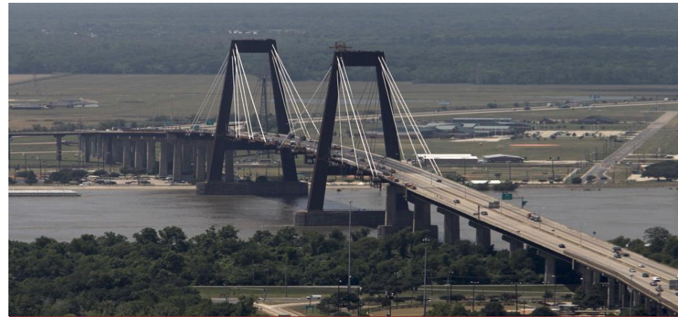
Merrick Creek Bridge Repair (USA)
