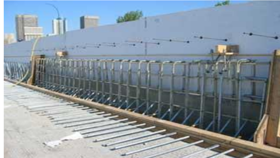
Bridge Barrier (Canada)
