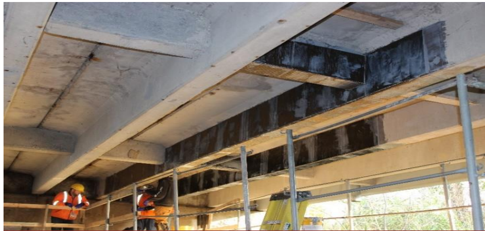
Merrick Creek Bridge Repair (USA)
