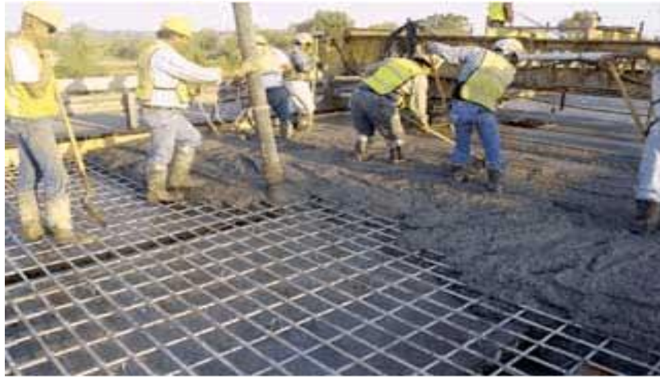
Bridge construction (Canada)
