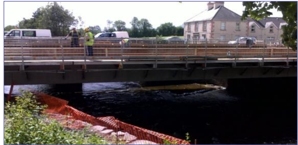
A new one-span bridge on a two-lane road of class A in Co. Fermanagh, Northern Ireland
