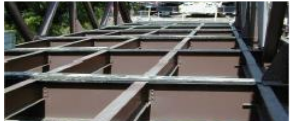
Repair of the Warren Farm Bridge in the village of Wellsburg, Chaemooon county, New York (USA)
